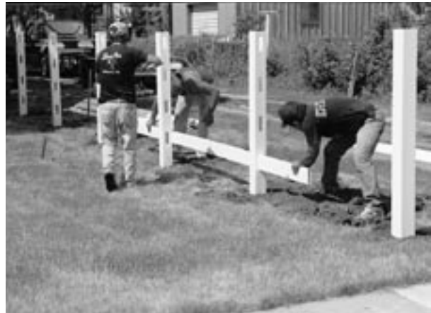
Threading the first rails, starting at the bottom. If spacing permits, rails are staggered at the joints.
