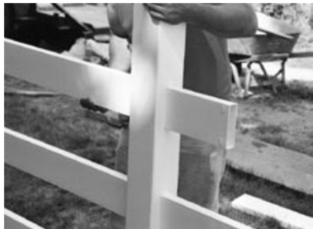
Rails are threaded through the pre-routed posts.
